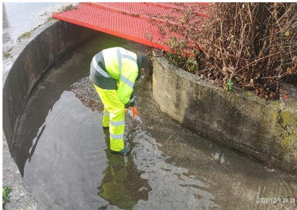
Figure 8: PVK storm water run-off sampling
